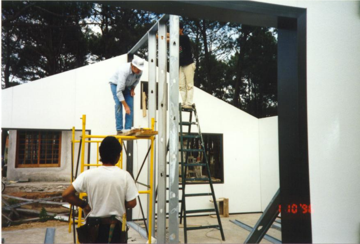
Hour 7 - Interior roof bearing wall is installed.
