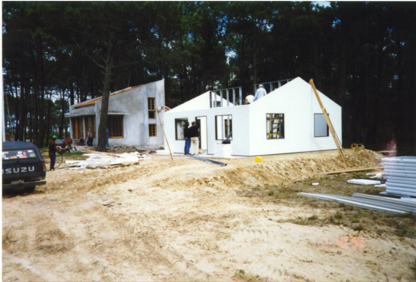
Hour 6 - View of completed exterior wall panels ready for roof panel installation.
