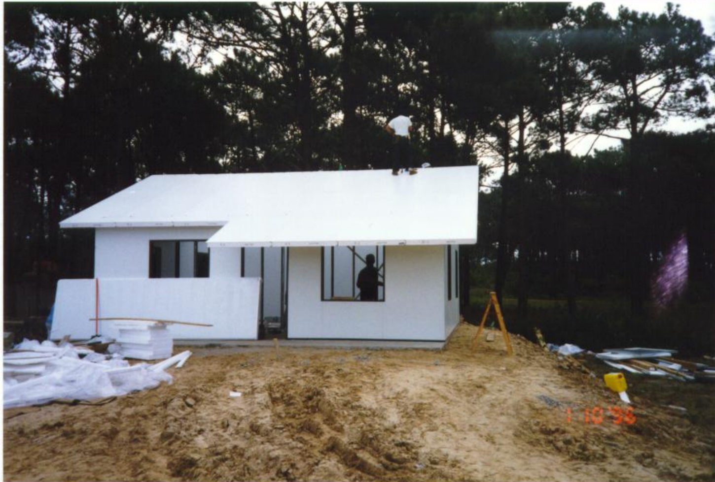
Hour 9 - Front roof panel installation is complete.
