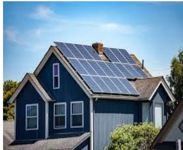
Solar Electric System / Batteries
