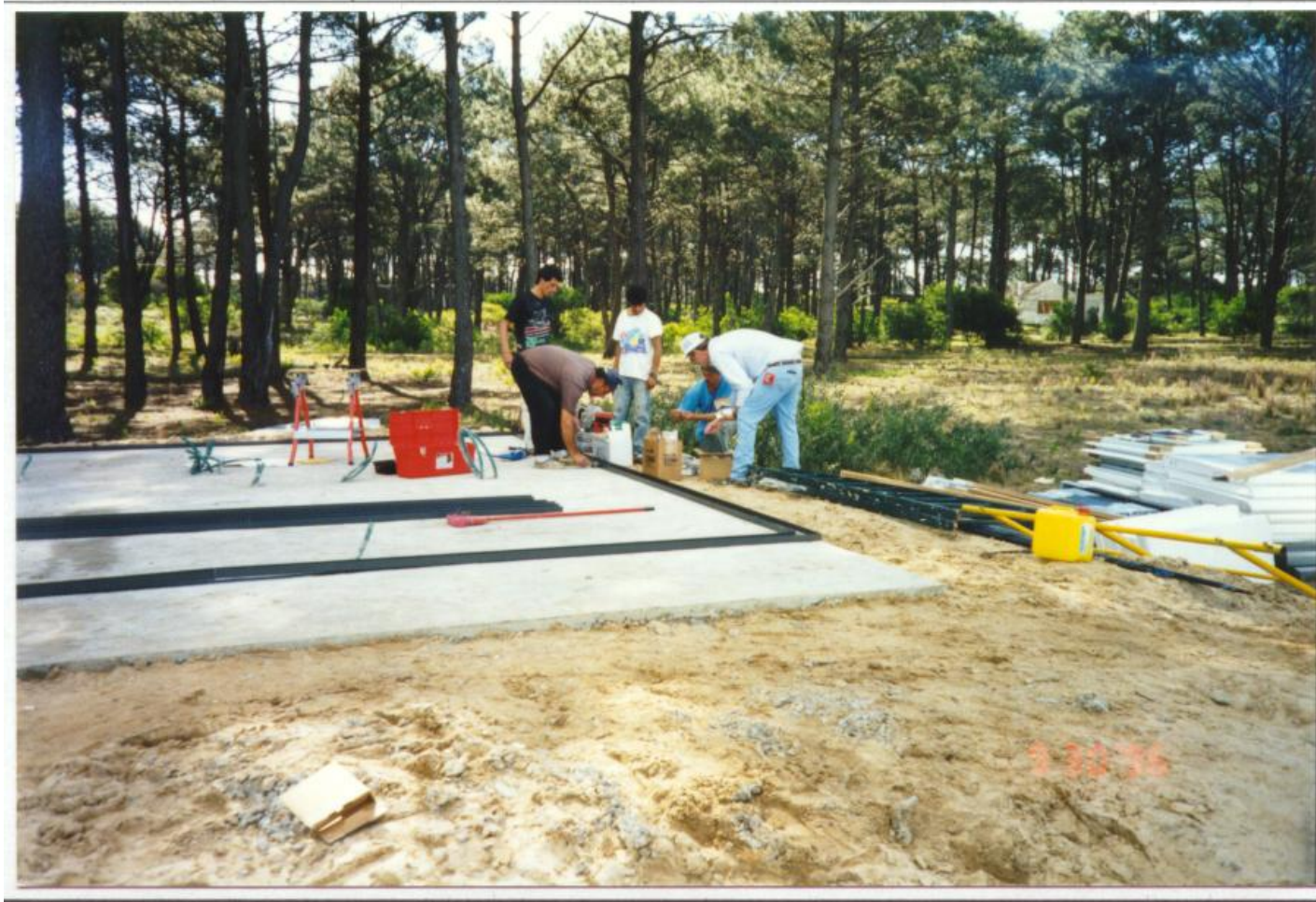
Hour 3 - Metal receiving track is attached to concrete foundation slab.
