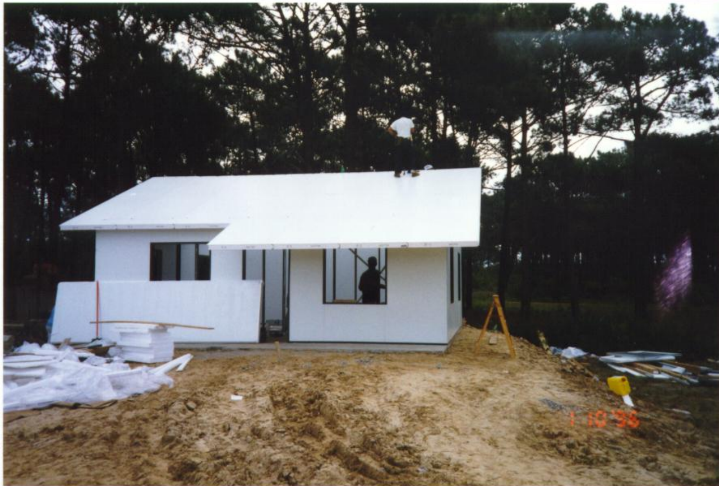
Hour 9 - Front roof panel installation is complete.
