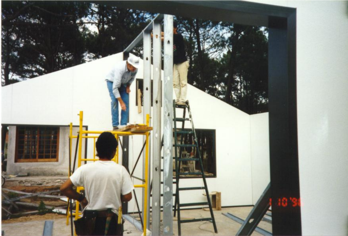
Hour 7 - Interior roof bearing wall is installed.
