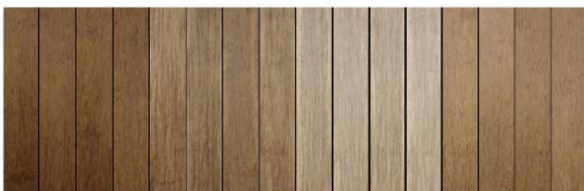
After Installation 2 Years After Use After Cleaning After Maintenance
