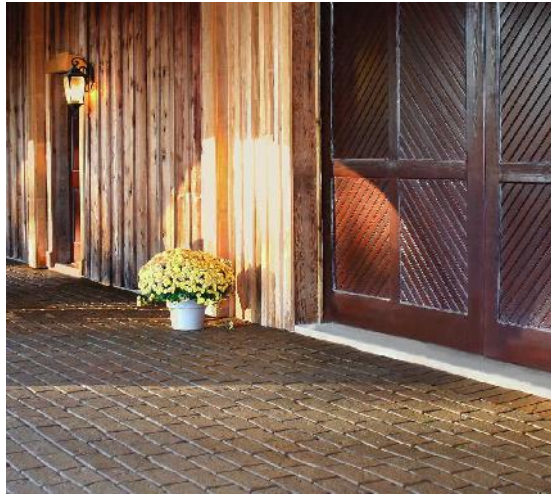
Photo of Rubber Cobblestone Pavers installed at Horse Barn for safety.
