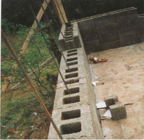
First Course of FASWALL Forms
