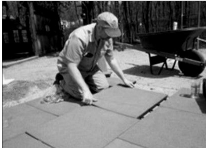
Playground Tile Installation
