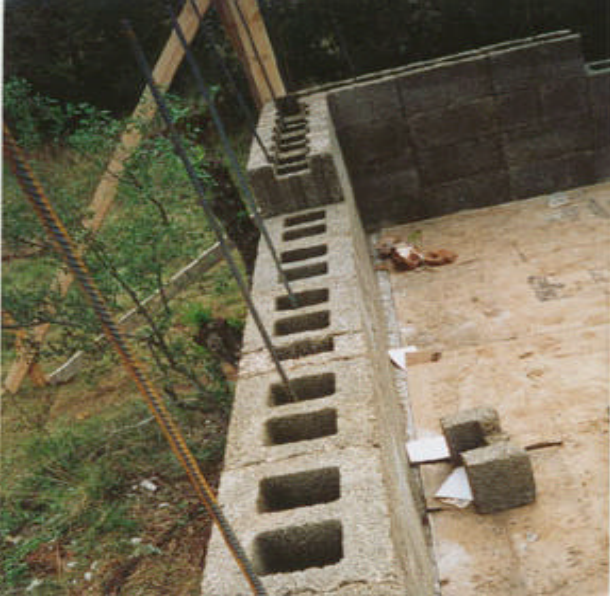
First Course of FASWALL Forms
