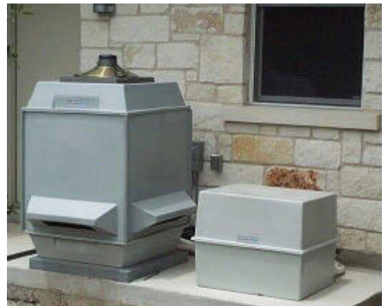
Condenser with Dual Compressor Box
