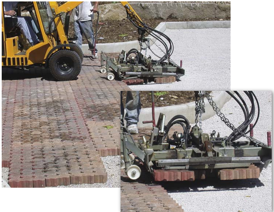
Figures 3 and 4. Permeable interlocking concrete pavement was mechanically placed over a 2 in. (50 mm) of chip gravel, a 4 in. (200 mm) thick base of No. 57 stone 5 in. (125 mm) thick No. 2 stone subbase.
