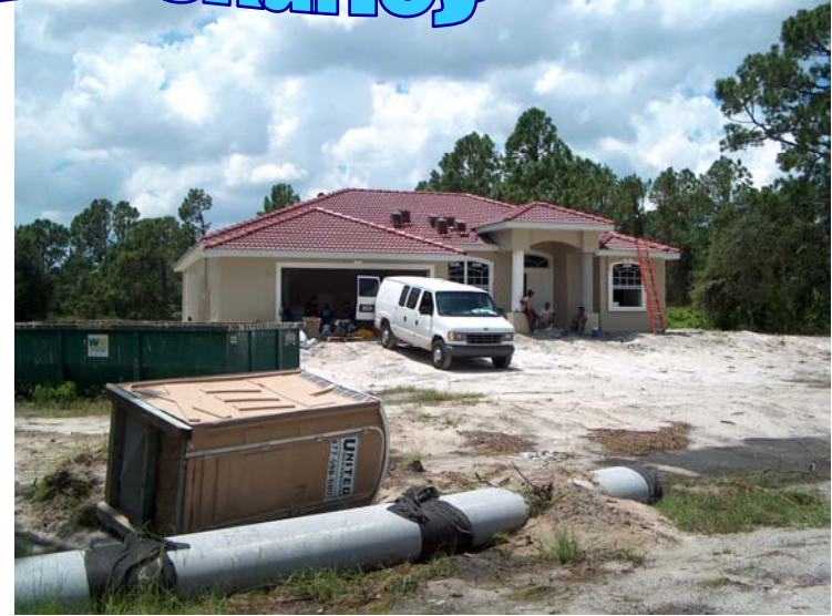
Morey's E-WALL home North Port, Florida
